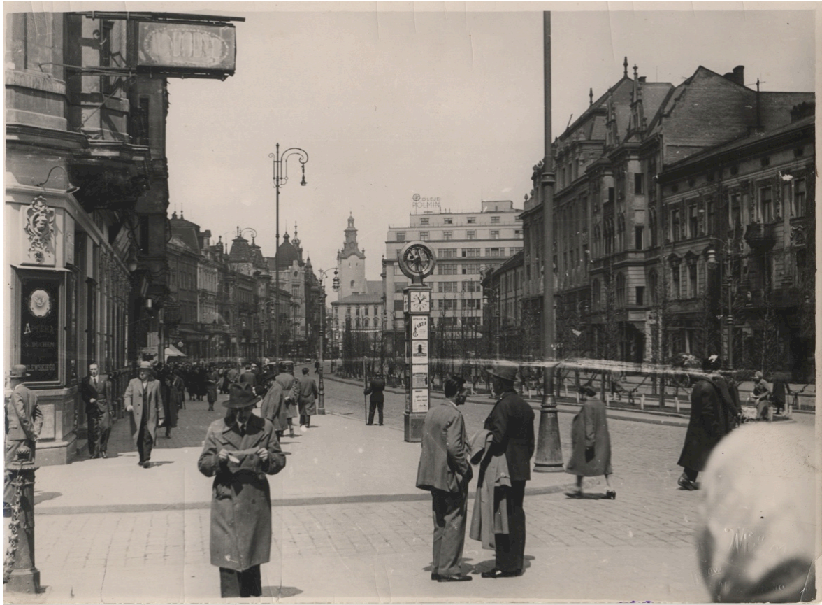
Fig.2. A view of Akademicka Street (today's Shevchenko Blvd.) in Lviv around 1930. At the end of the boulevard—the modernist building built by Ferdynand (Feiweł) Kasler for Jonas Sprecher in 1928-1929. Source: Marek Münz, photo 13x18 cm., Lviv Historical Museum.
