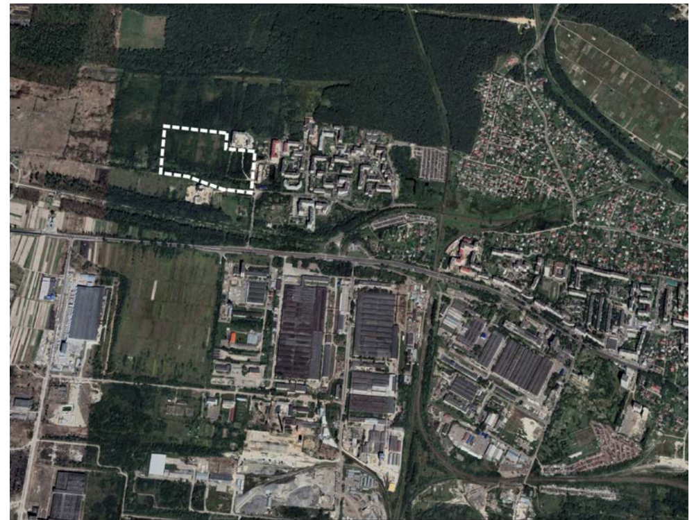
Fig. 05 Ryasne neighborhood & surrounding I Source: Lviv City Council Office of Urban Planning / Google Earth
